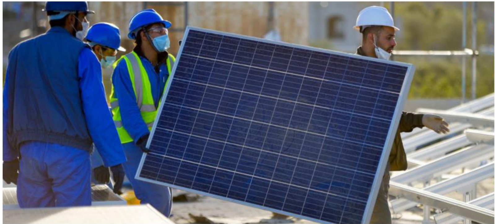
UNDP Yemen | Men install solar panels for a hospital in Yemen.
